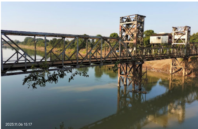
Dikhous Steel Bridge; Image Credit: Dilip Changkakoty
